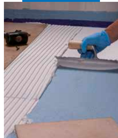
Bonding tiles on Mapelastac AquaDefense
