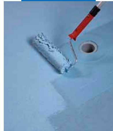
Application by roller of Mapelastac AquaDefense second coat
