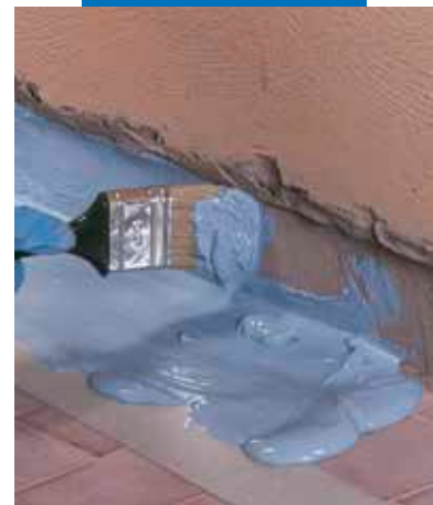
Application of Mapelastac AquaDefense by brush between floor and wall before applying Mapeband
