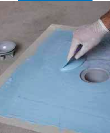
Impregnating Drain Vertical fabric with Mapelastick AquaDefense
