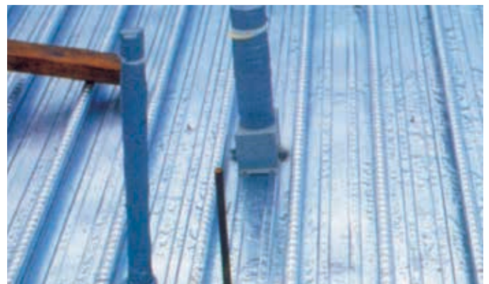
Step 6: Cut penetration.
