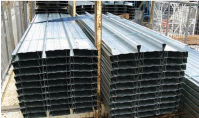
Step 1: Open BONDEK® sheet bundles.
