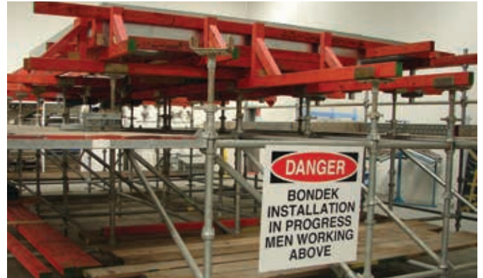
Step 2: Place props if required.
