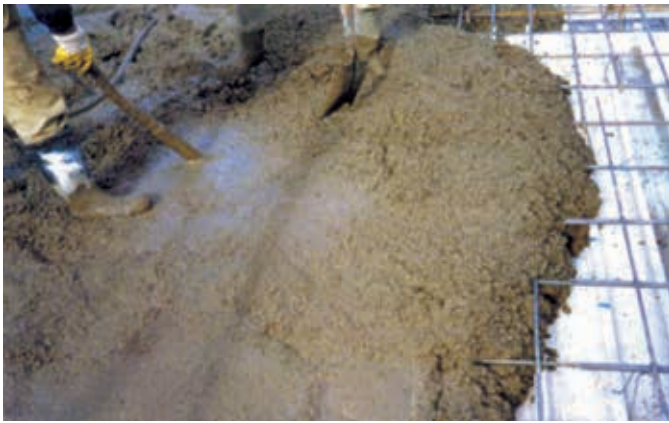
Step 8: Place concrete.
